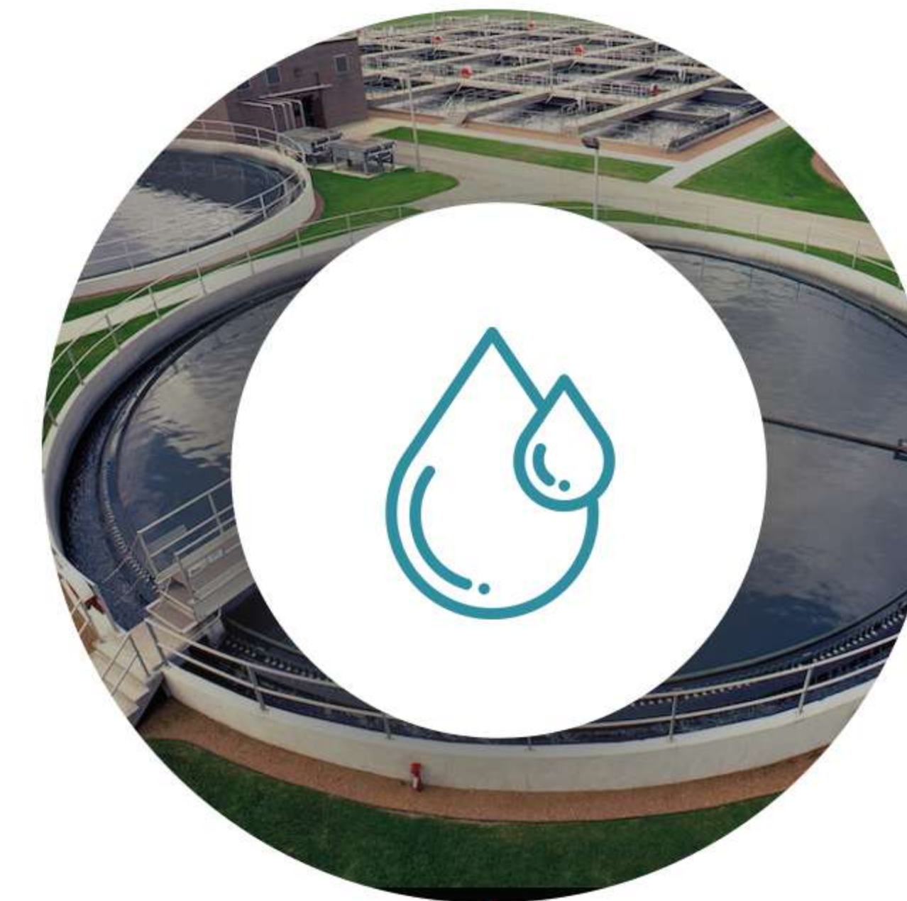
2. Water Treatment Systems
