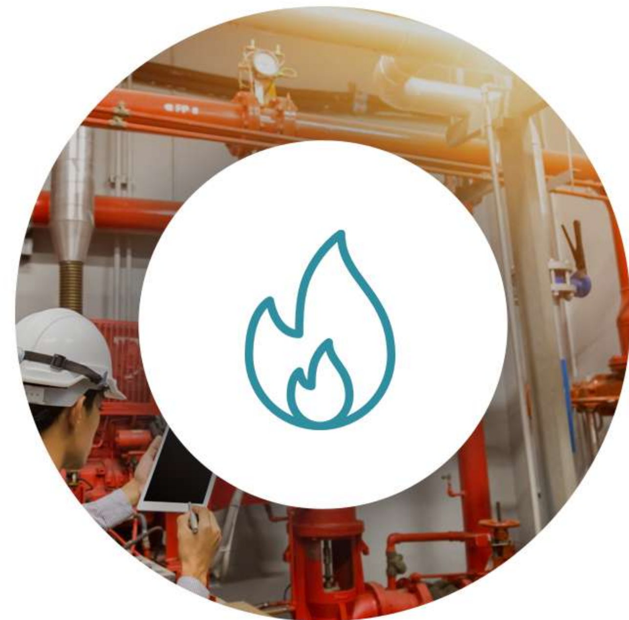
1. Fire Safety Systems
